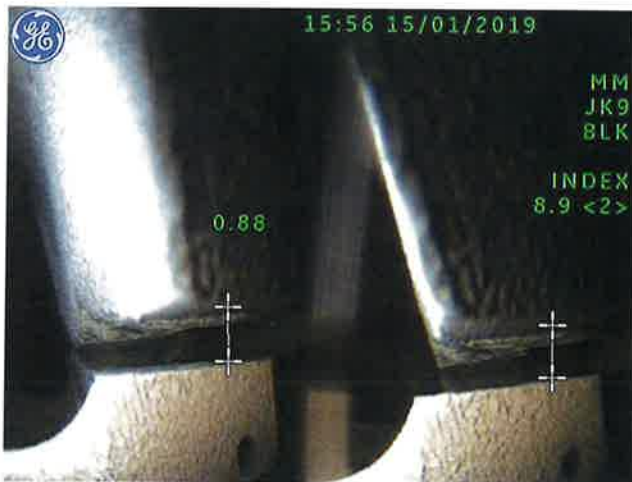
Gap with no erosion
