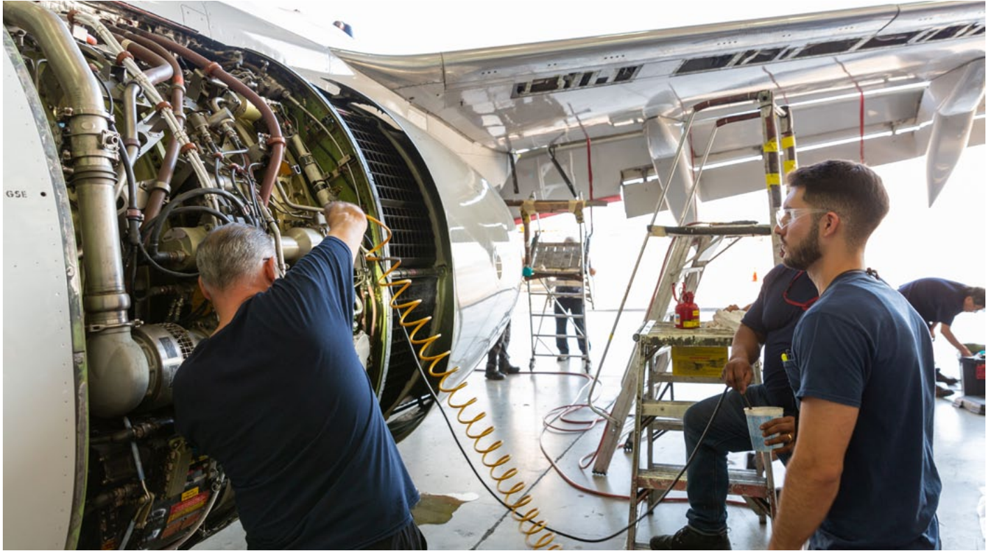
Technician shortages are most noticeably in North America. © AAR
